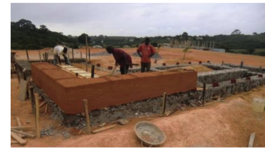
RAMMED-EARTH WALL ON SITE
